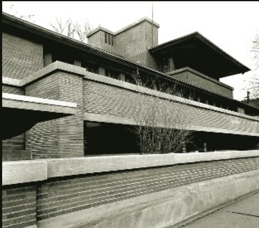
The brickwork (FLWFDN)
