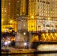
The four bridge houses provide a canvas for bas-relief sculptures depicting pivotal moments in the city's history.
